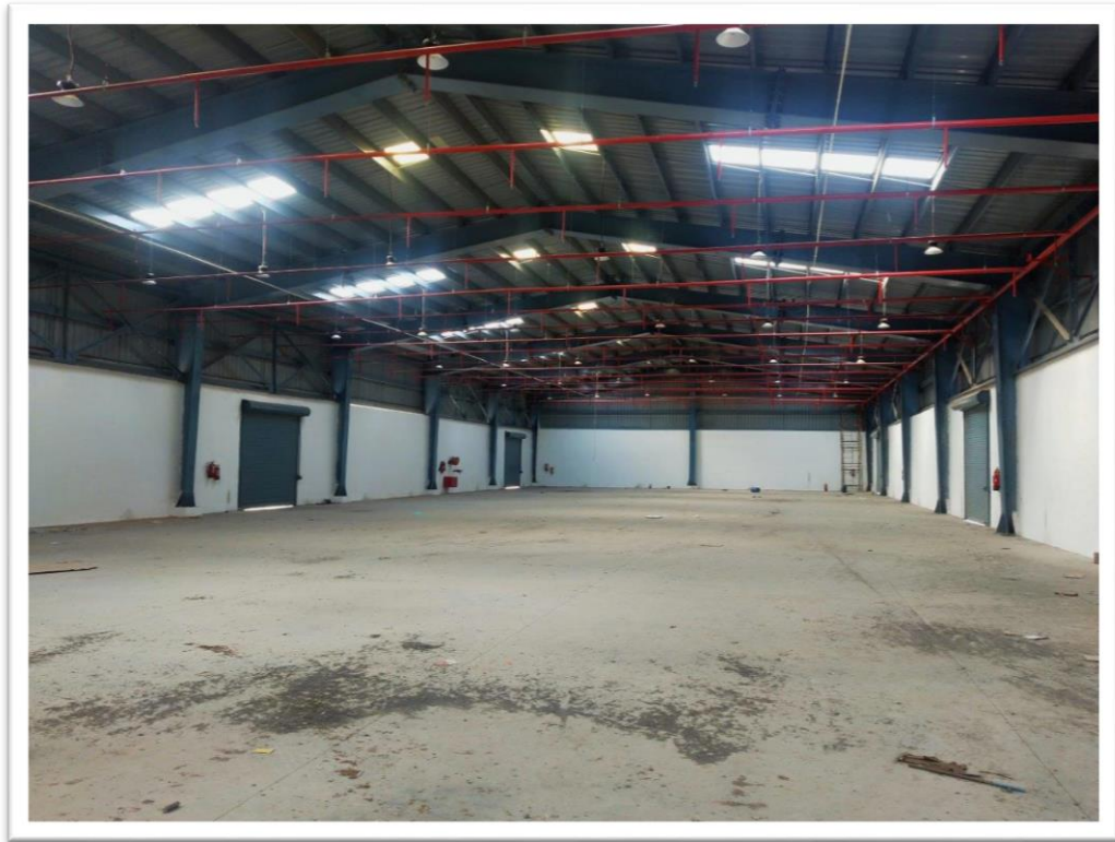
Figure -8 : Fire Sprinklers
