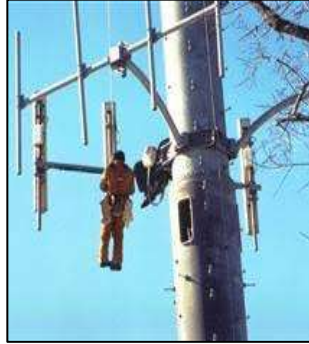
Figure-1.5 Rigger attached with truck crane and hoist
