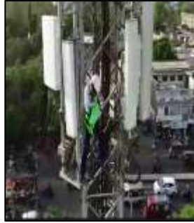
Figure-1.8 Maintenance on top of four-legged tower
