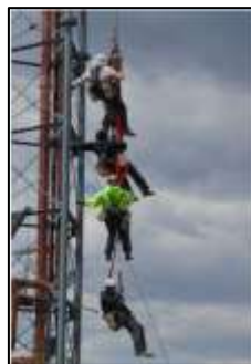
Figure-1.3 Maintenance work performed by riggers
