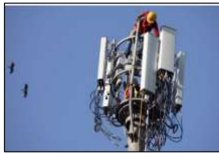
Figure-1.2 Tower Rigger
