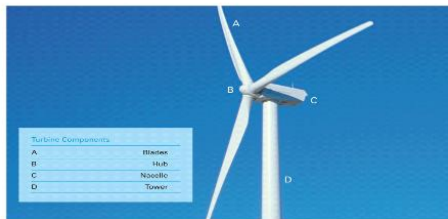
Figure 1.2: Turbine components
