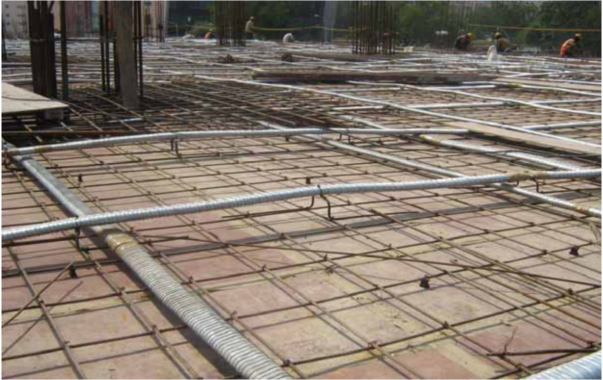
Fig. 8.5 Tendon duct and chair provided for eccentricity
