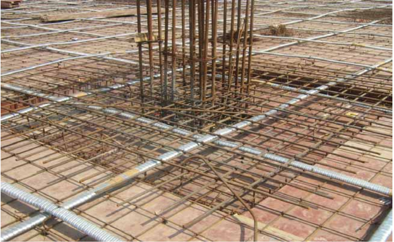
Fig. 8.7 Reinforcement at the drop panel
