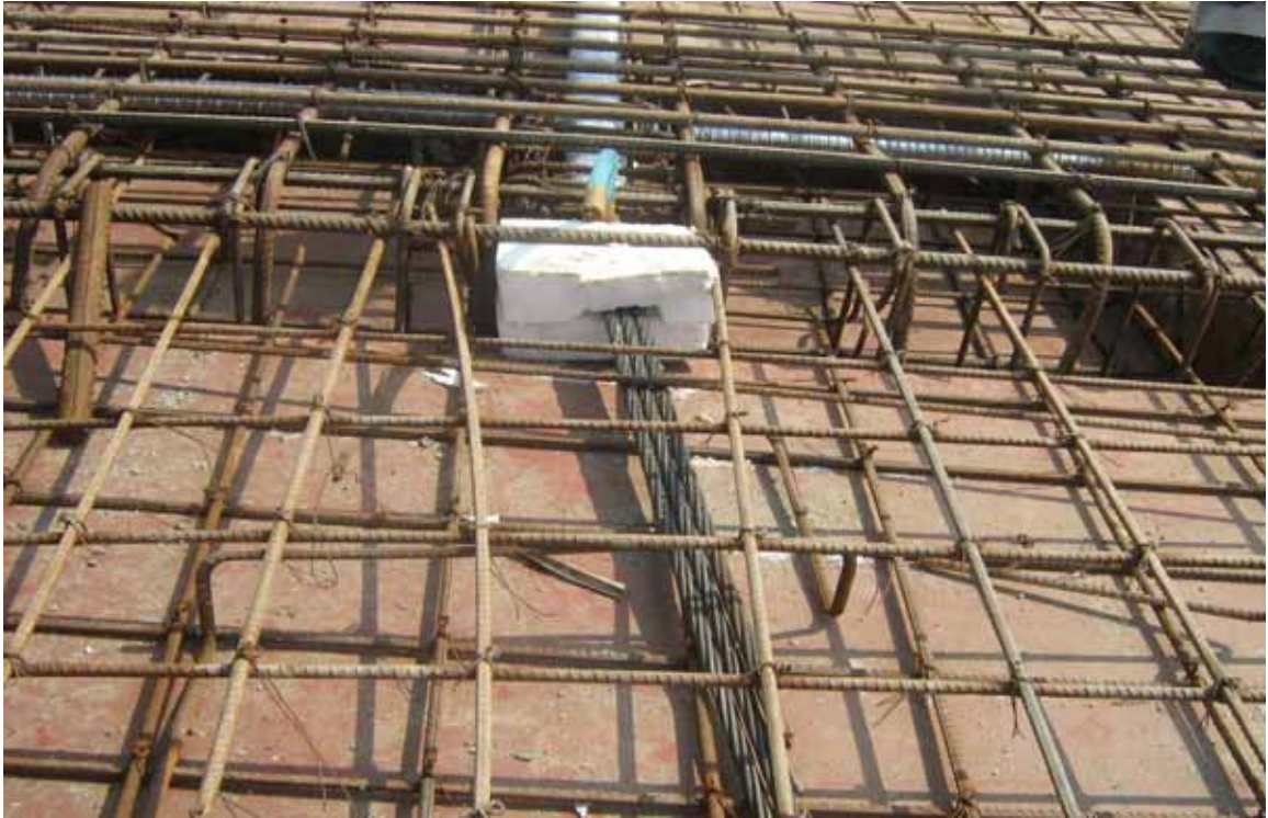
Fig. 8.1 Stressing end for the cables
