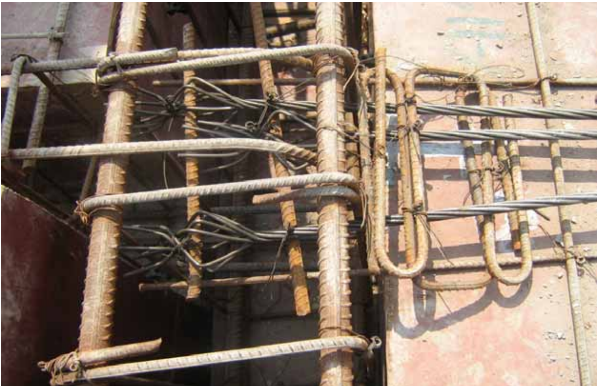
Fig. 8.6 Dead end and beam reinforcement
