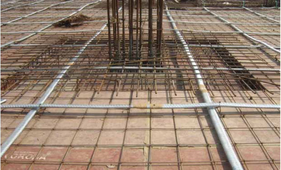
Fig. 8.3 Laying out tendon and the drop panel reinforcement
