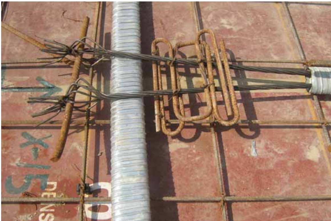
Fig. 8.2 Guide ring, balloon and anchorage for the cables
