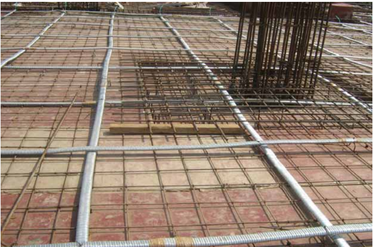
Fig. 8.4 Placing of tendon and slab reinforcement
