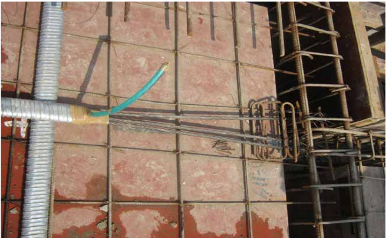
Fig. 8.8 Vent pipe provided for grouting
