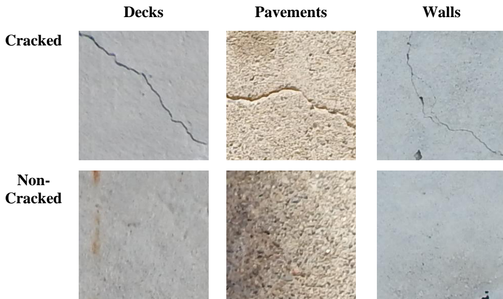
Figure 30 Sample images from SDNET dataset. (Structural Defects Network (SDNET) 2018)
