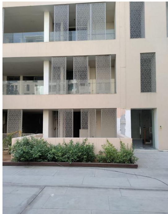
Fibre jaali on balconies
