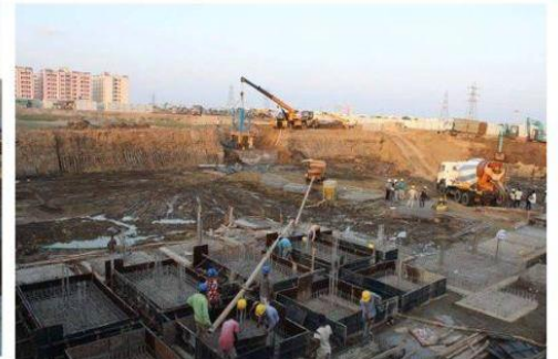
3. FIGURE 22 ND SHUTTERING AND REINFORCEMENT WORK FOR FOOTINGS SOURCE : AUTHOR
