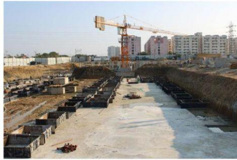
2. FIGURE 21 ST PCC AND SHUTTERING FOR FOOTINGS SOURCE : AUTHOR
