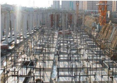
4. FIGURE 23RD CASTING OF FOOTINGS SOURCE : AUTHOR
