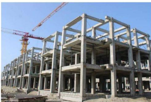
10. FIGURE 28TH ERECTION OF BEAMS, COLUMNS AND SLAB IN UPPER FLOORS SOURCE : AUTHOR
