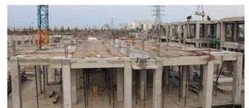
9. FIGURE 27TH MONOLITHIC RCC FRAME AFTER SCREED CONCRETE AND WET JOINTING OF BEAM, COLUMN AND SLAB SOURCE : AUTHOR
