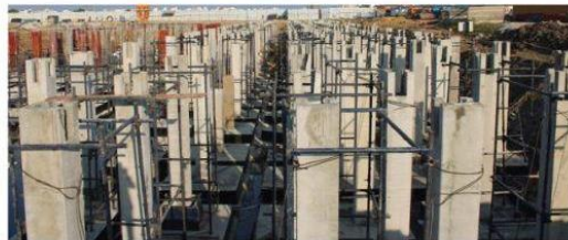
5. FIGURE 24TH ERECTION OF PRECAST STEM COLUMNS FROM FOOT- INGS SOURCE : AUTHOR
