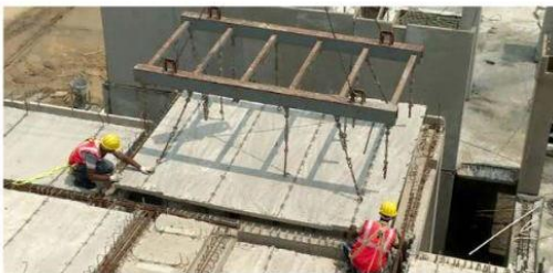
7. FIGURE 26TH PLACEMENT OF PARTIALLY PRECAST SLAB SOURCE : AUTHOR
