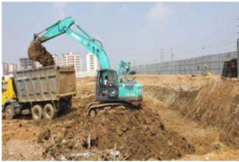
1. FIGURE 20TH EXCAVATION WORK FOR FOUNDATION SOURCE : AUTHOR
