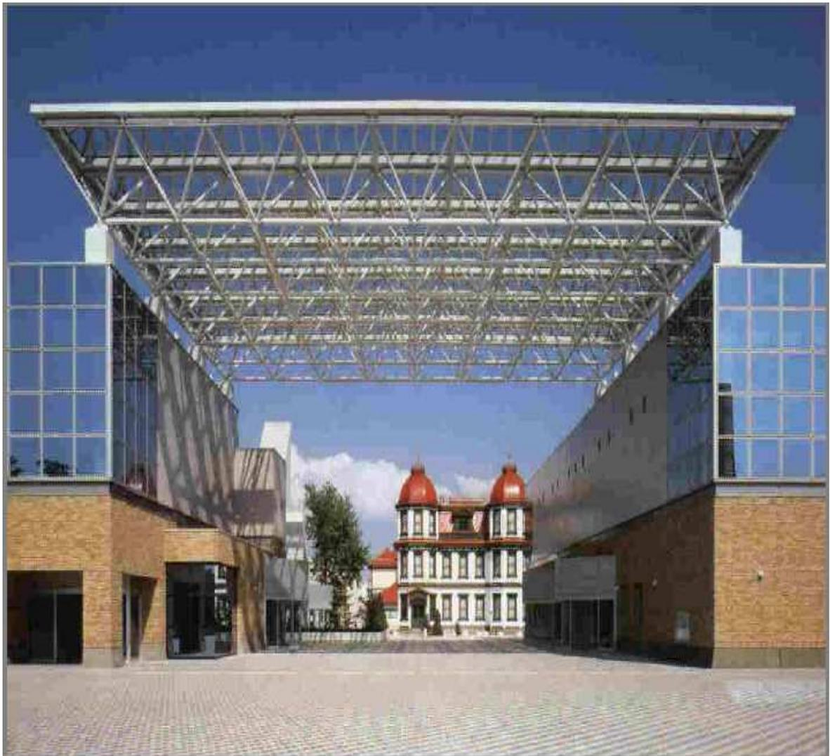
Figure 1.3 Double layer grid
