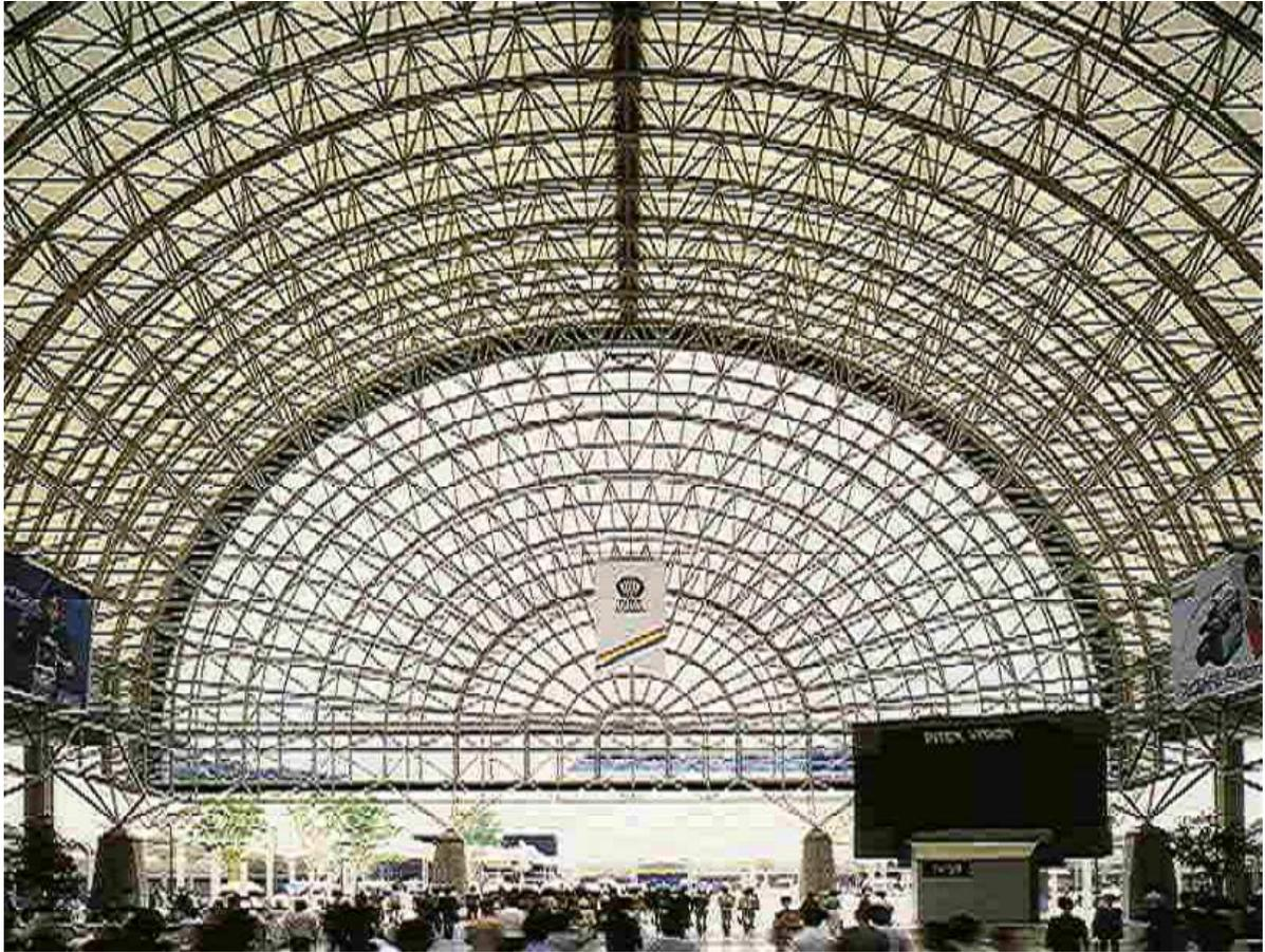
Figure 1.5 Braced folded structure- Braced barrel vault
