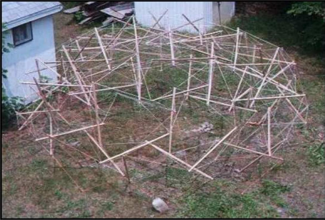
Figure 1.9 Double layer tensegritic dome
