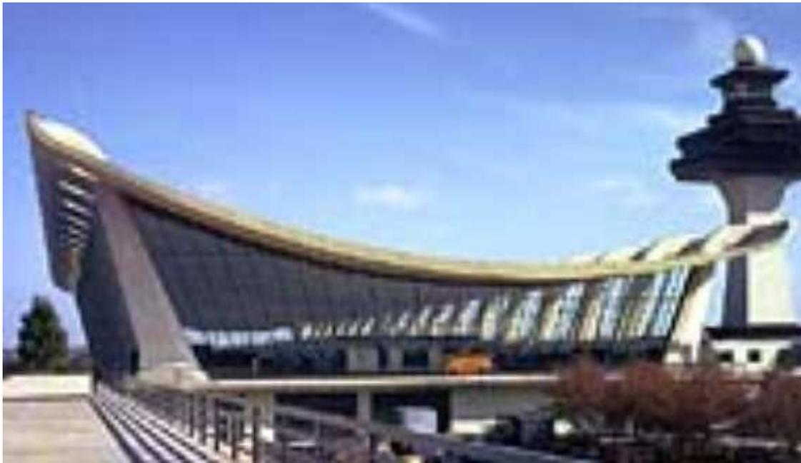
Figure 1.6 Cable suspended roof structure
