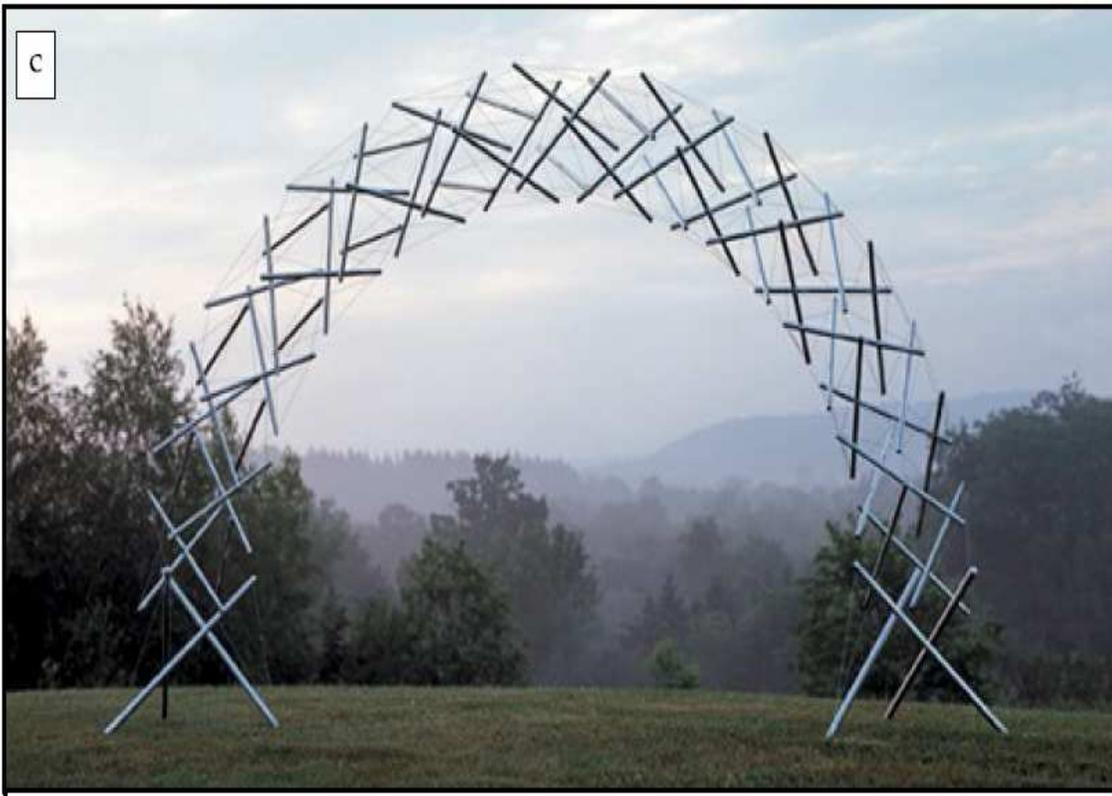
Figure 1.10 Tensegritic arch
