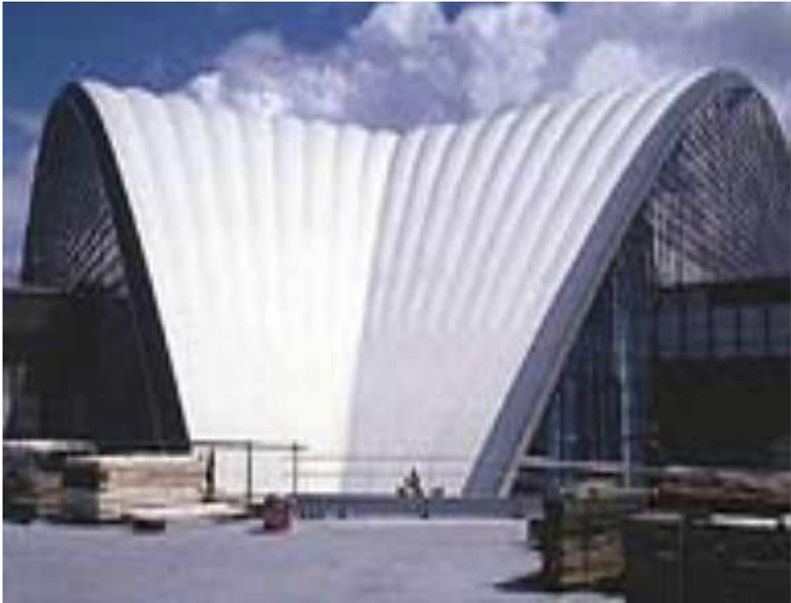
Figure 1.4 Braced dome structure
