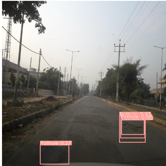
Figure 4.17: Pothole Detected in Real Time
