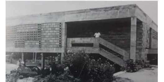
Fig. 8.2.16: Concrete frame structure with pre-cast blocks in-fill wall at the Pressure Transducer Unit Source: (Prakash, 2012 p.84)
