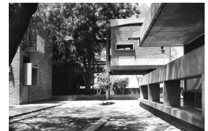
Fig 3.7: : Exposed brick and concrete structure Source: © Kanvinde Rai & Chowdhury
