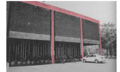
Fig 8.2.10: Front Elevation of the Museum of Life and Evolution; Illustration showing the uninterrupted columns, extending to the roof Source: (Bhatti, 2018 p.264) – Diagram by the author
