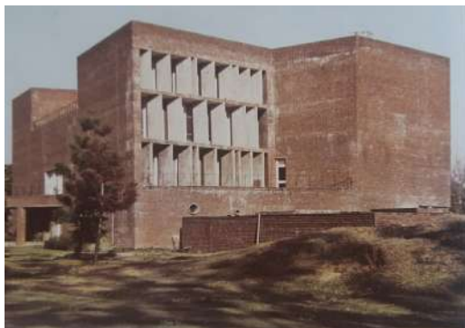
Fig 8.3.44: Concrete louvers at U.T. Guest House Source: (Prakash, 2012 p.50)
