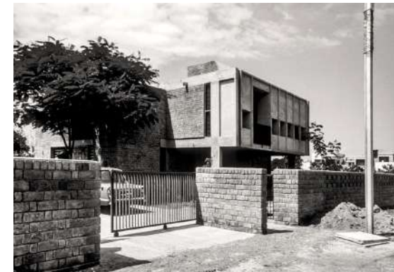
Fig 3.4: Image showing the separation between the wall and the column. The image also shows the concrete façade of the residence. Source: HCP official website
