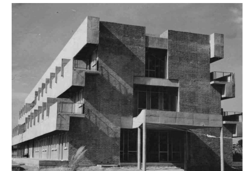
Fig. 8.2.2: Front elevation showing section of the concrete elements used i.e. beams and slabs. The front porch is also in exposed concrete. Source: SDSA Website
