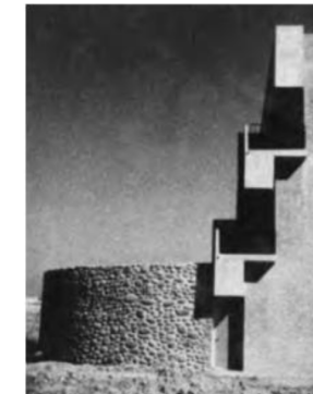
Fig8.2.1. The random rubble stone curvilinear walls for the cafeteria Source: (Prakash, 2012 p. 28)
