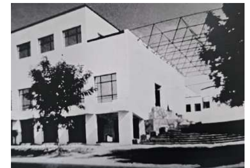
Fig. 8.3.34: Space frame at the entrance of the DLF Shopping Arcade
