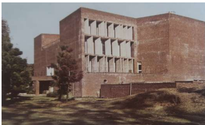
Fig 8.2.8: Concrete louvers at the U.T. Guest house, solid monolithic brick facade Source: (Prakash, 2012 p.50)
