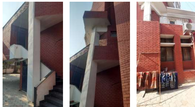
Fig 8.4.10: Images showing the column on the façade, appearing and moving into the building as the plan changes Source: Photos by the author
