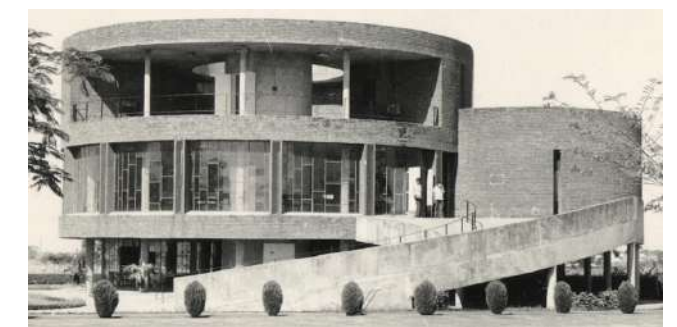
Fig. 8.1.16: View of the CSIO Canteen, showing the open façade with undulatory glazing Source: SDSA Website
