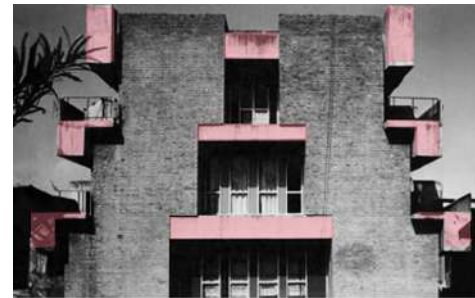
Fig. 8.4.1: Elevation of the building showing the enlarged concrete beams Source: (Prakash, 2012 p. 28) – Diagram by author
