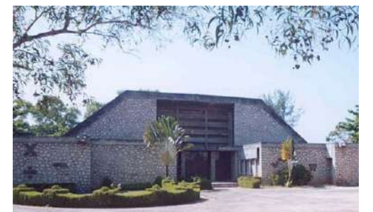
Fig 8.2.18: The VSSC Central School made with stone rubble masonry, with a concrete roof Source: ©MATTER 2014
