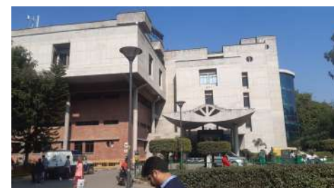
Fig. 8.1.31: Front elevation of the Advanced Eye Care Center, PGIMER, showing the upper floors projecting outwards, supported by columns Source: Photo by the author
