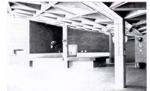
Fig. 8.4.13: Image showing the waffle slab used at the Vikram Sarabhai Hall in Ahmedabad Source: (Prakash, 2012 p. 70)
