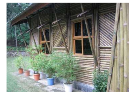
Fig. 8.2.32: Use of bamboo to create structural members, covering walls and frames for windows Source: TheBetterIndia (Menon, 2017)
