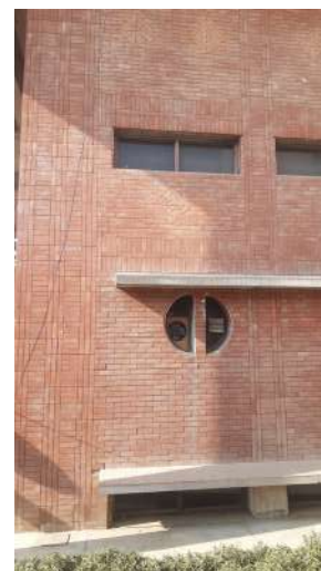
Fig. 8.2.29: Patterns formed by brick tiles on the front façade Source: By author
