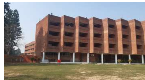
Fig 8.3.6: Elevation of the U.T. Guest House in brick, lifted on concrete columns; monolithic and solid forms. Source: Photo by author
