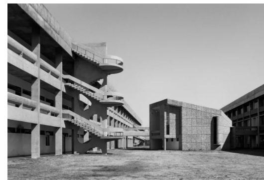
Fig 3.10: Exposed concrete free standing staircase at IIT Delhi Source: Madan Mahatta Archives, PHOTOINK
