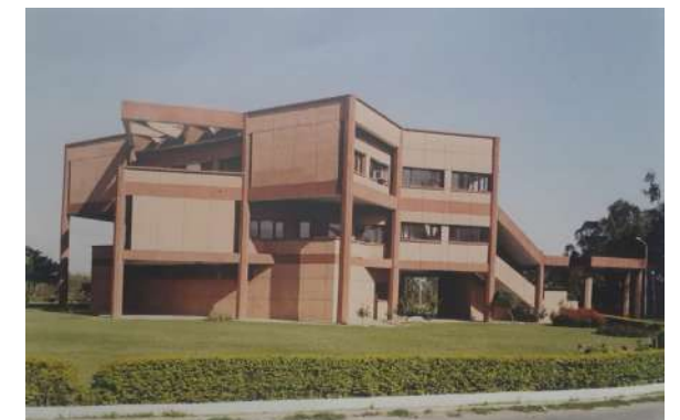
Fig. 8.2.26: Stone cladding on the Administration building at NIPER. The darker stone gives an expression of a frame structure and the light stone of an in-fill wall Source: (Prakash, 2012 p. 122)
