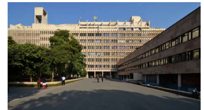
Fig 3.11: Image showing the vertical concrete louvers on the façade Source: https://www.photoink.net
