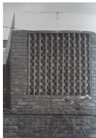
Fig. 8.2.23: Use of brick jali wall in Dr. Amod Gupta's Residence Source: (Prakash, 2012 p.164)
