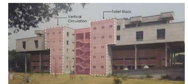
Fig. 8.3.55: Image showing the service block in the Elevation at Advanced Eye Care Center Source: (Prakash, 2012 p.103) – Diagram by the author
