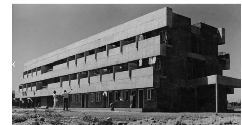
Fig. 8.2.3: Side elevation shows the concrete parapet, which gives the impression of large beams. Source: ©MATTER 2014
