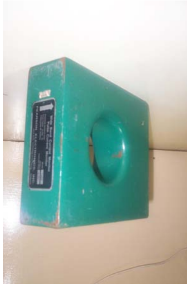
Figure 6.10.3 Current Transformer (1000:1)
