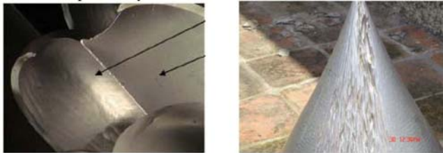
Fig. 9: Erosion of bucket (left) and needle (right)
