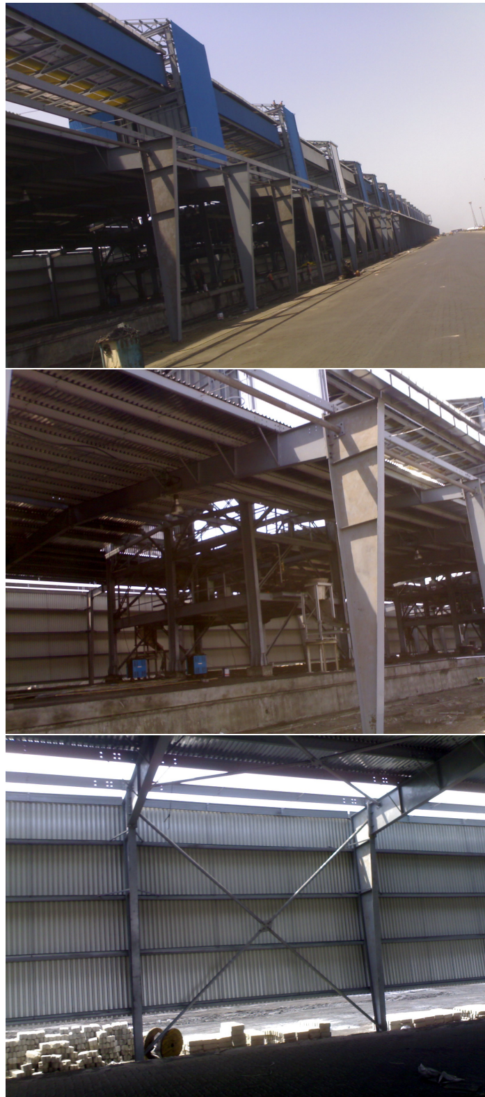
Figure 7.2: Side View of F.C.C ware house, Portal Section, Portal Bracing
