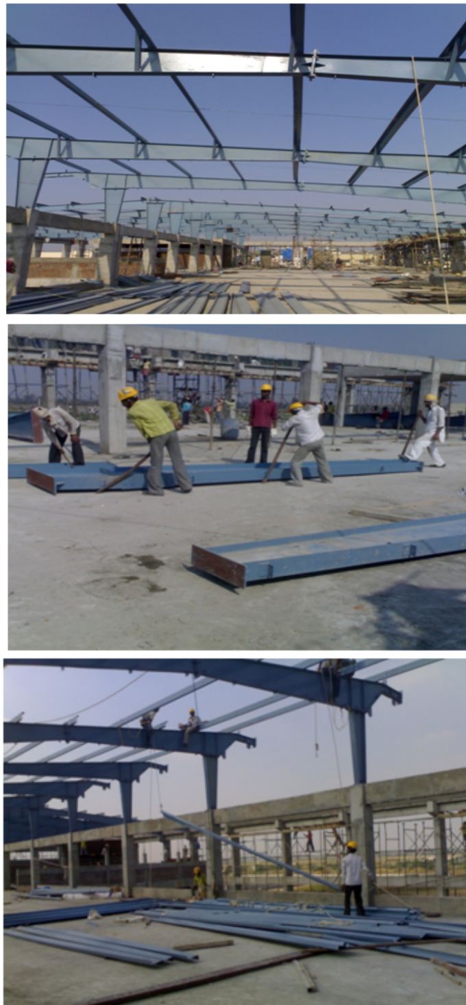
Figure 7.1: Front View of the Building (30m), Transport the section to required location, Placing the Z-Purlin on Rafter
