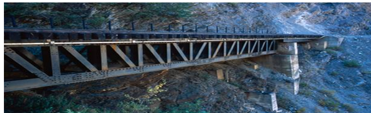
Figure 3.4: Typical Truss girder
