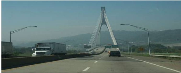
Figure 3.21: Inverted V-type pylon
