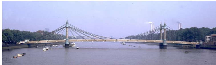
Figure 3.6: Albert Bridge, London fan type arrangement
