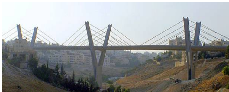
Figure 3.20: Y-type pylon
