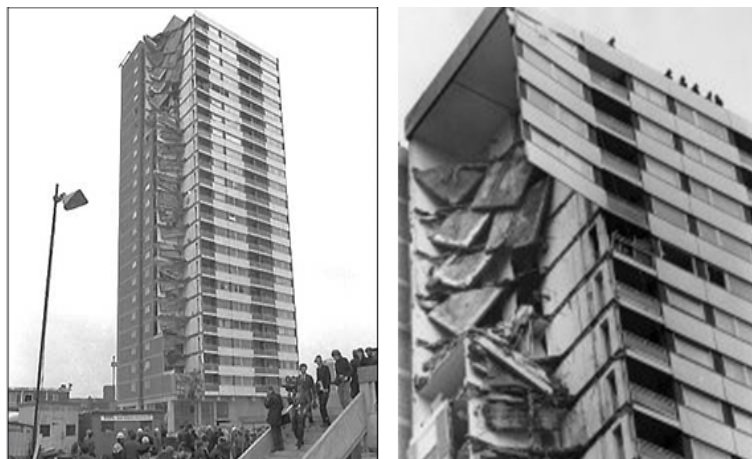
Figure 1.3: Collapse of Ronan point apartment
