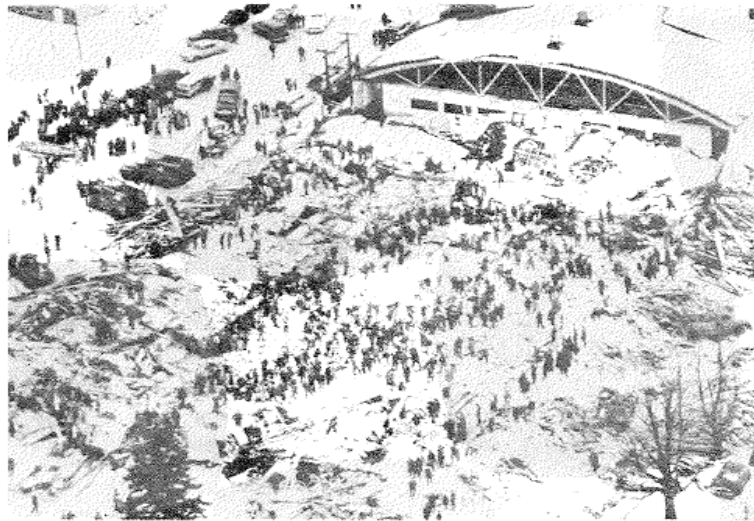
Figure 1.4: Collapse of arena under snow load
