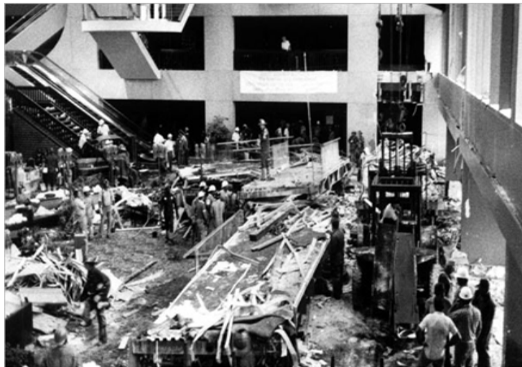
Figure 1.7: Collapse of Hyatt Regency Hotel
