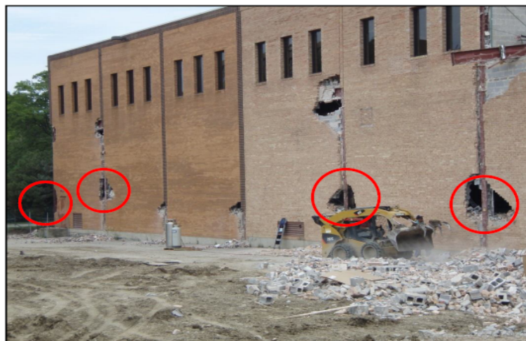
Figure 1.11: The circled columns were removed for experiment
