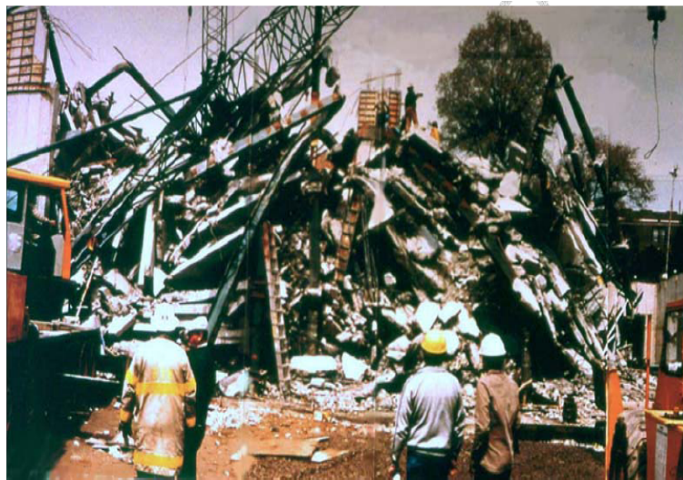
Figure 1.8: Collapse of L'Ambiance plaza
