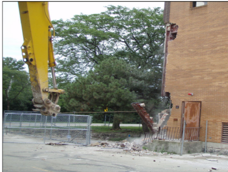
Figure 1.12: Torched section of column being removed
