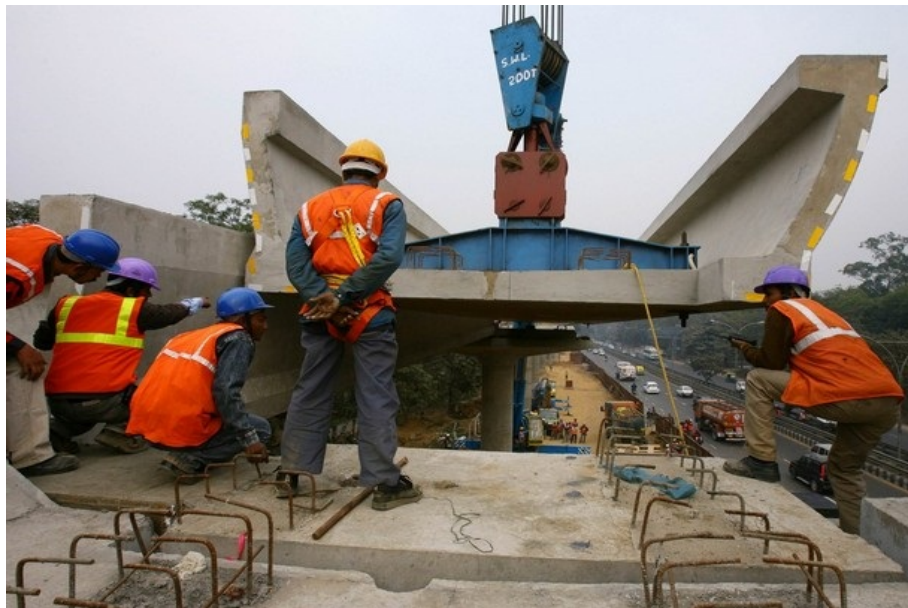
Figure 1.9: Erection of U-shaped girder
