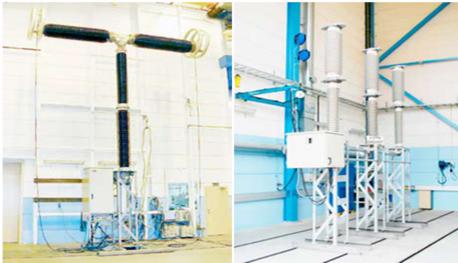
Figure 3.3: Test of circuit breakers at laboratory [1]
