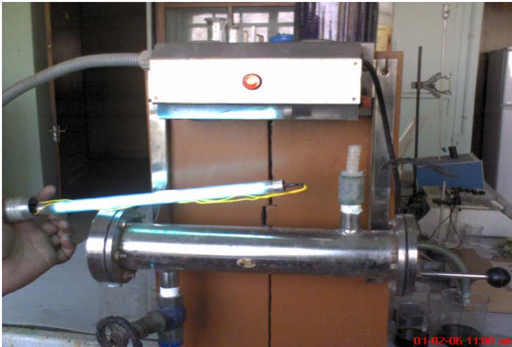
Figure – 3.1.1 Ultra Violet Lamps in running condition
