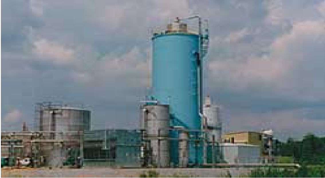
Fig: 6.2 Photo of a BIOPAQ IC reactor at a Kraft pulp mill in the USA
