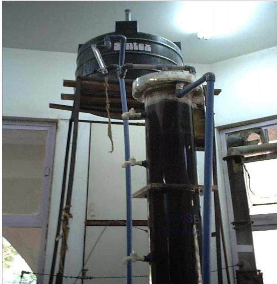
Figure: 7.1.1. Influent collection system
