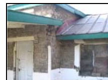
Fig. 18 Stone Masonry walls
