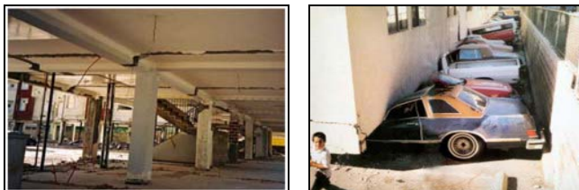
Fig. 4 Picture showing soft storey
