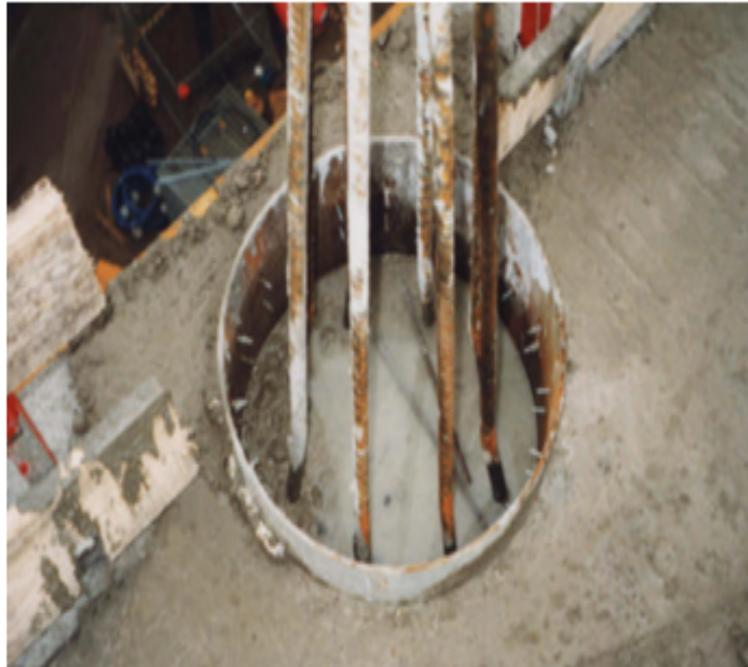
Figure 1.16: Tubular Column With Nails as Shear Connectors and Reinforcement on Site (Citibank Duisburg, Germany)
