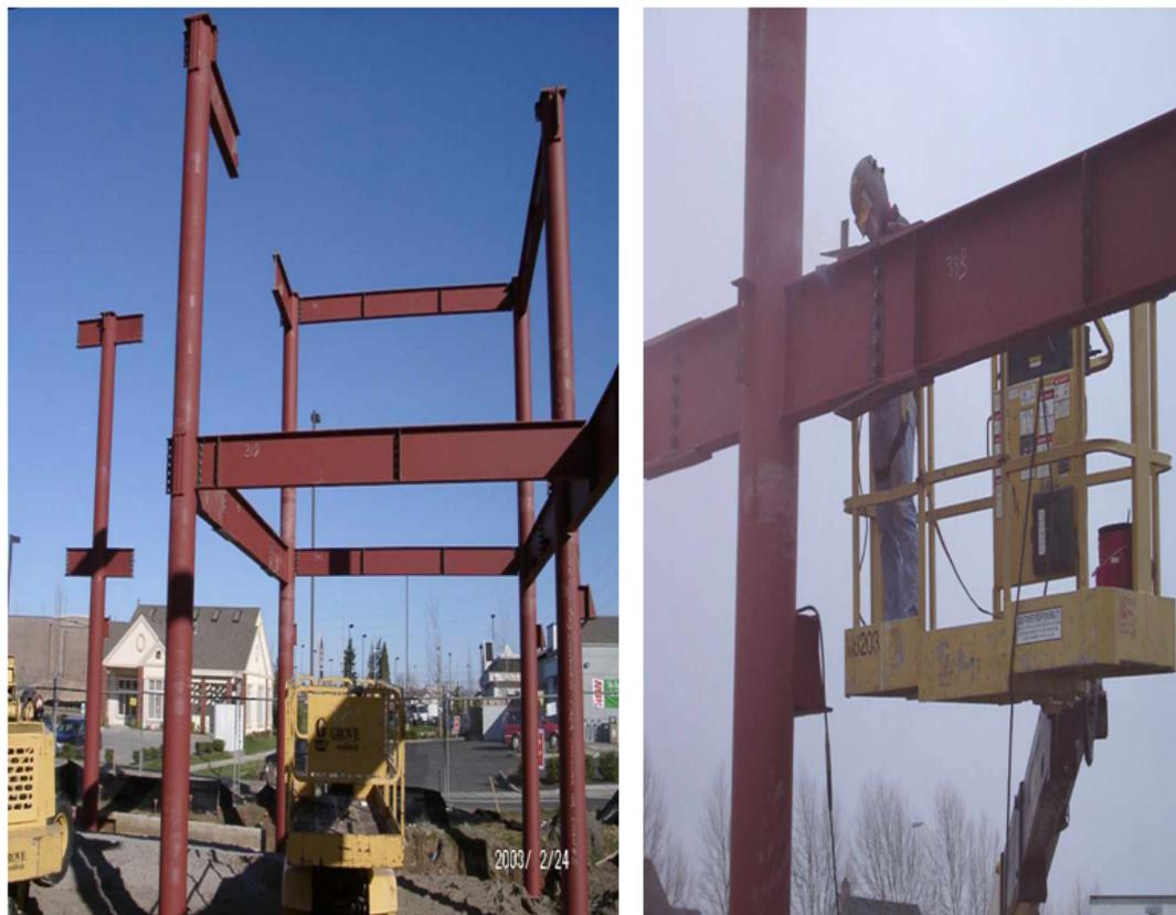
Figure 3.6: Shop-fabricated CFT Joint
