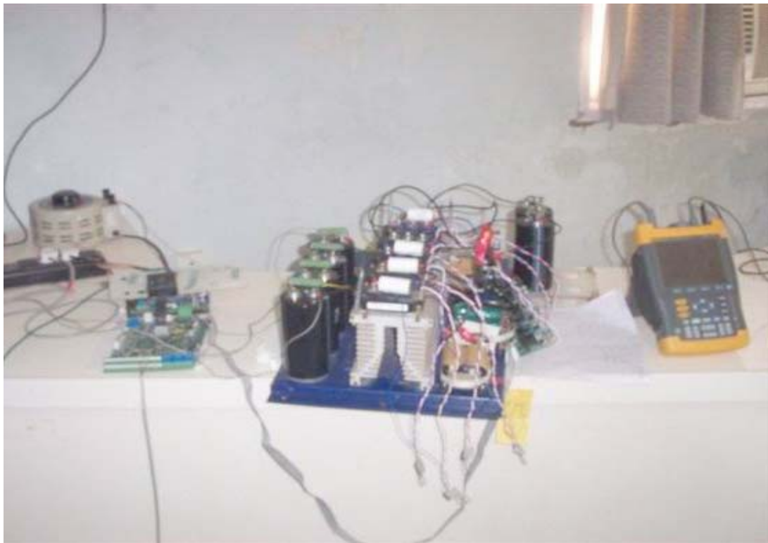
Hardware set up for isolated high power converter module
