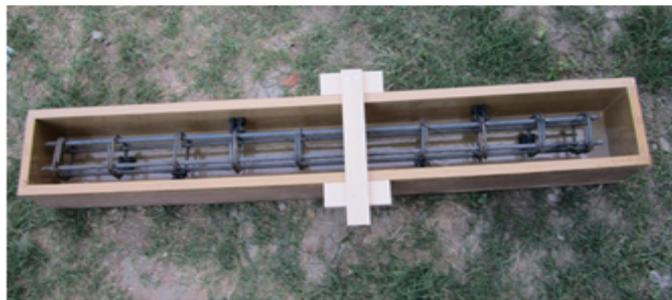
(a) Formwork for sharp edges
