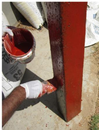
(c) Application of one coat of saturant
