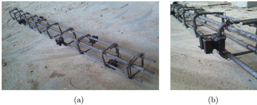
Figure 4.2: Reinforcement cage for columns with PVC cover
