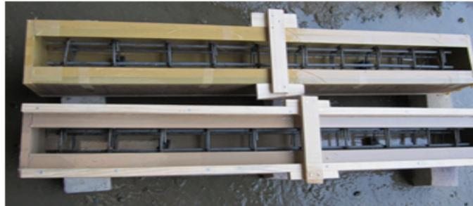
(b) Formwork for different corner radii
