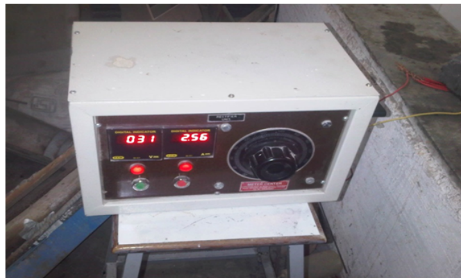
Figure 3.23: Rectifier for DC power supply
