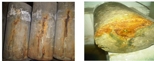
Figure 4.16: RC specimens after cracks and corrosion started
