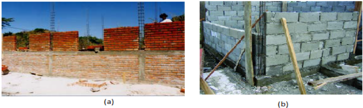
Figure 2.7: confined masonry construction
