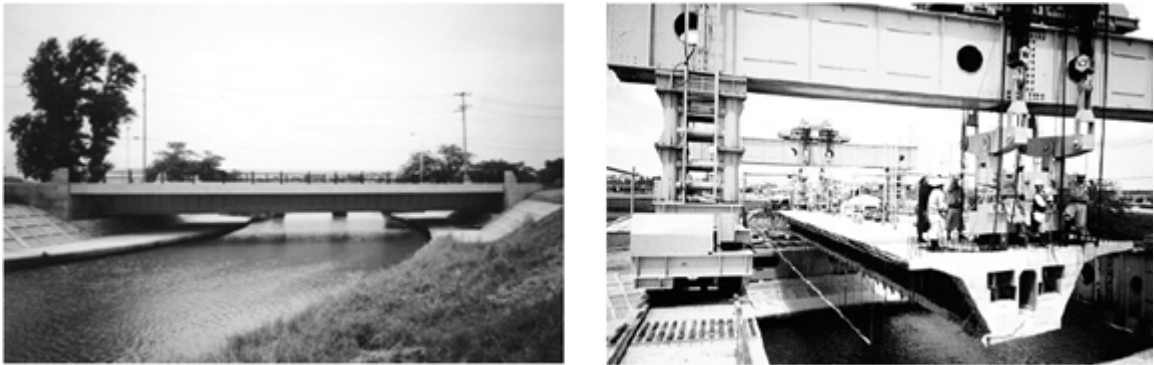
Figure 1.10: Shinkai Bridge (a) completed and (b) during erection
