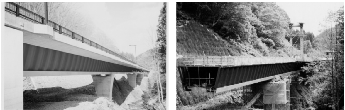
Figure 1.11: Ginzan-Miyuki Bridge (a) completed and (b) during erection
