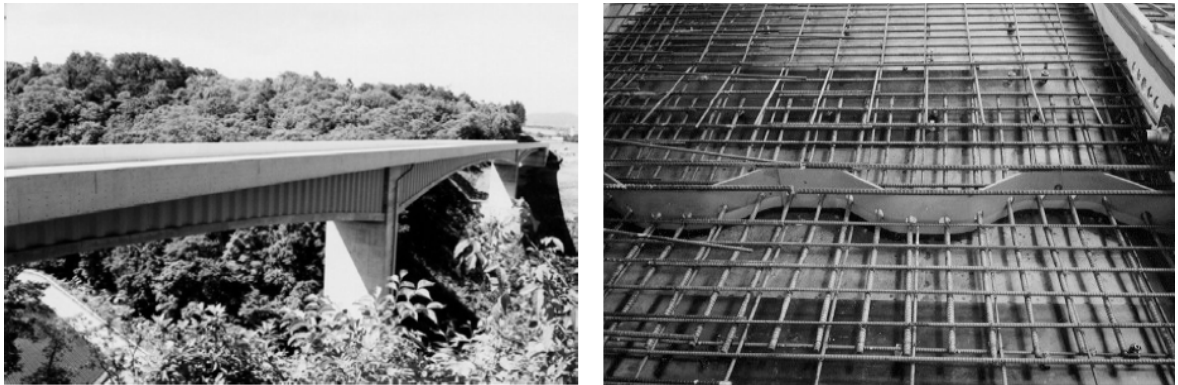
Figure 1.12: Hondani Bridge (a) Completed and (b) Embedded Connection
