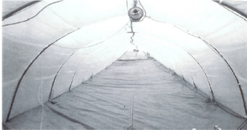
Figure 1.9: The inside of the collector tunnel with the stainless steel bows the poly-ethylene cover hemi-spherical and the black plastic sheet in the bottom[3]
