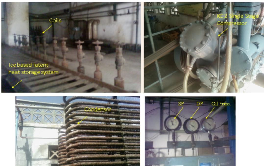
Figure 4.11: Ice based latent heat storage system, compressor, condenser and pressure gauges
