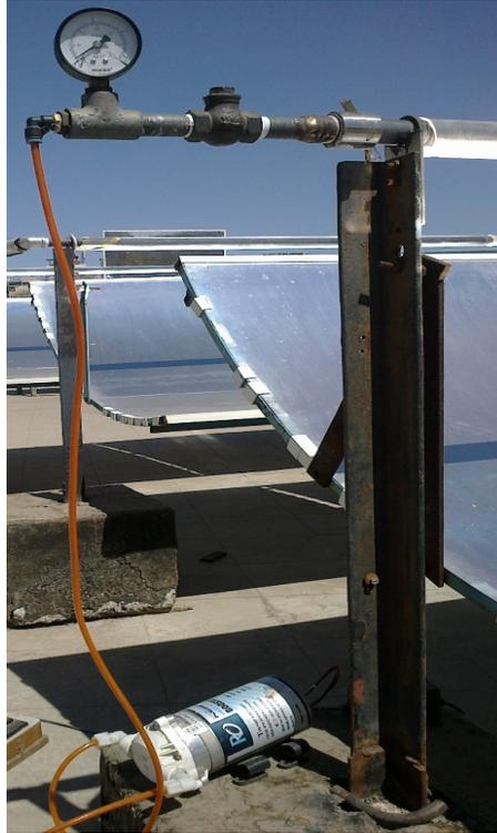
Figure 4.2: water inlet to PTC using pump
