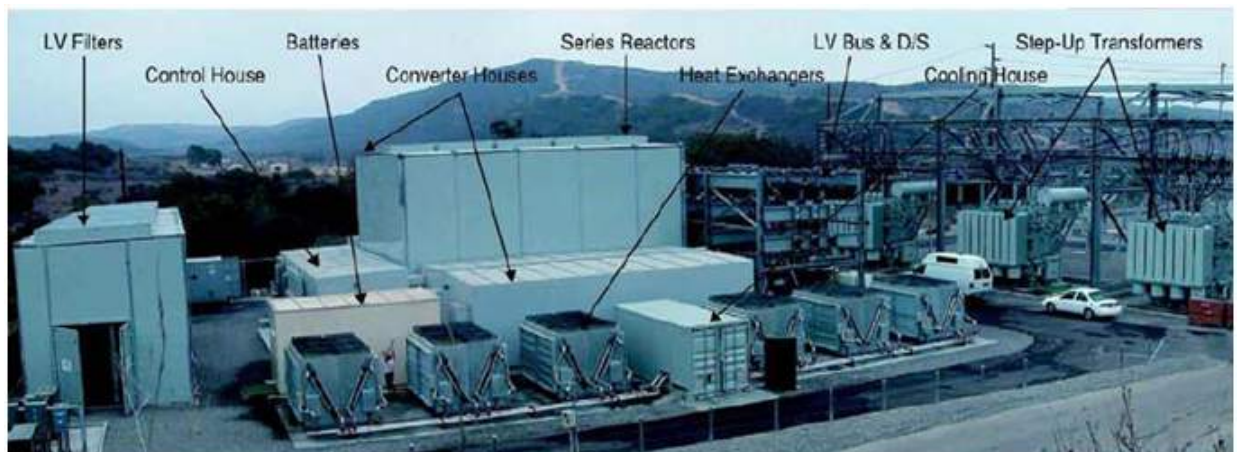
Figure 3.14: External view at Talega
