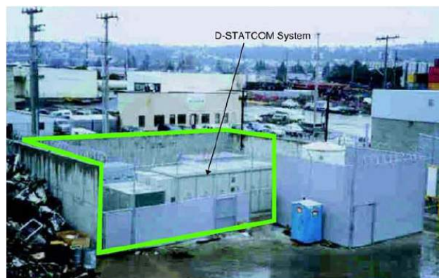
Figure 3.16: External view at steel recycle facility
