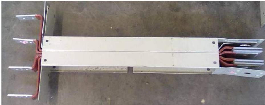
Figure 5.6: Existing Low voltage sandwich bus duct
