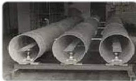
Figure 1.3: Isolated Phase Bus Duct
