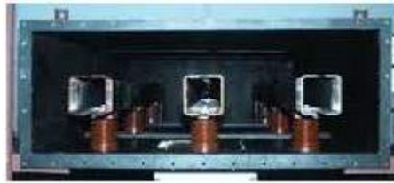
Figure 1.2: Non Segregated Phase Bus Duct
