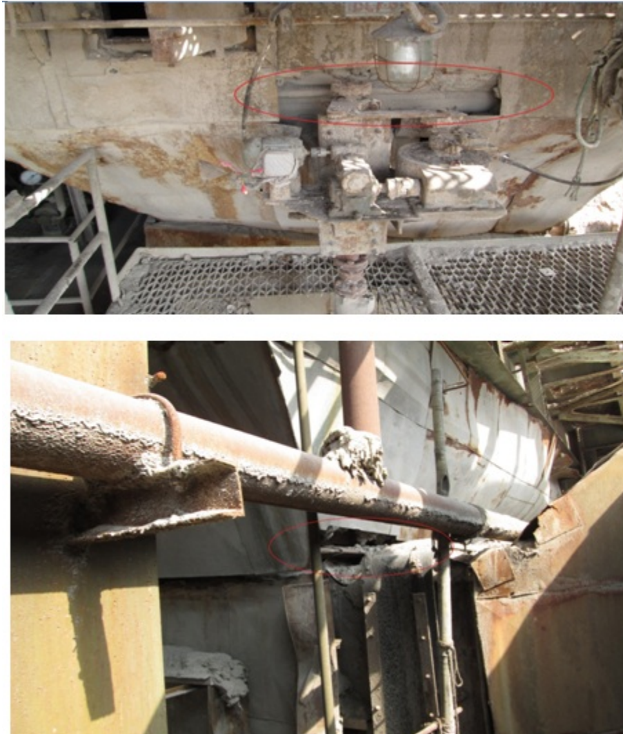
Figure 4.7: Insulation of APH
