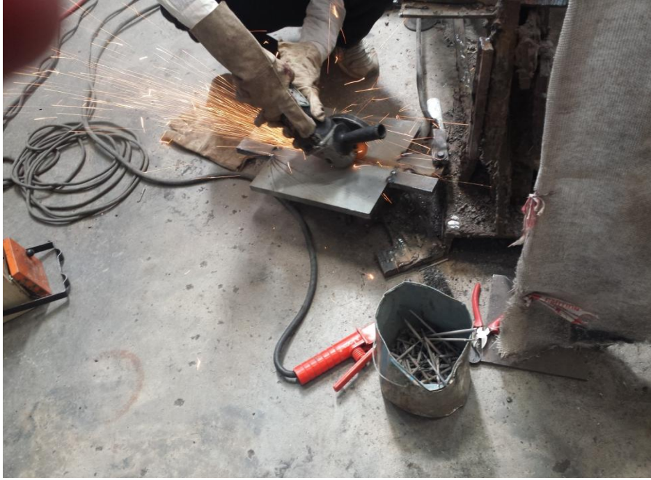
Fig.7 grinding after root pass and prepare for the hot pass
