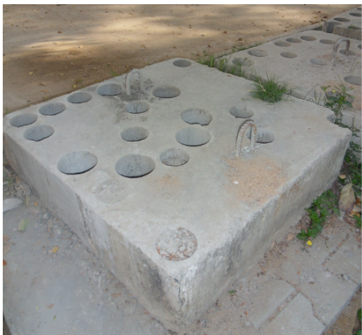
Figure 4.13: slab panel after extraction of core
