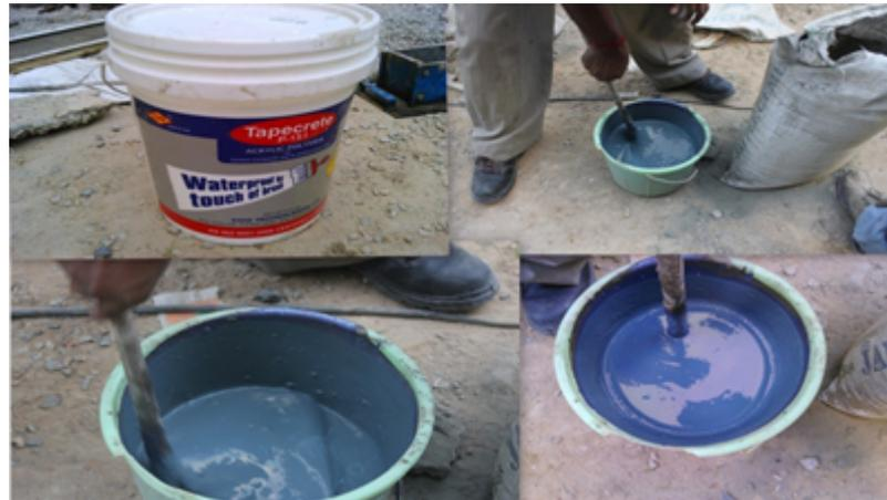
Figure 3.16: Preparations of Polymer Grout
