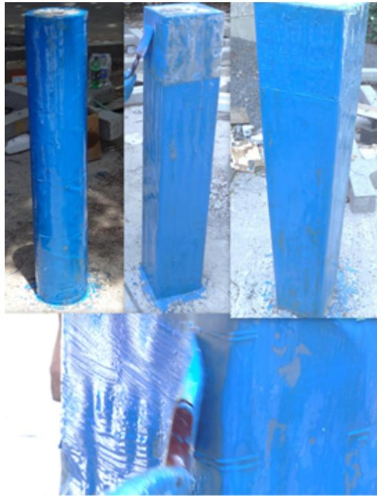
Figure 3.27: Application of Final Coat
