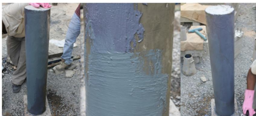
Figure 3.17: Applying First Coat
