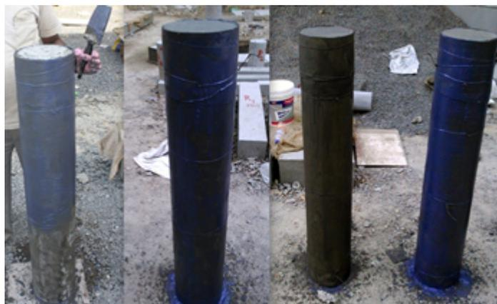
Figure 3.19: Applying Final Coat on Column
