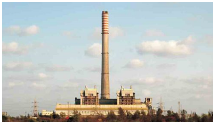
Figure 1.4: Multi Flue RCC Chimney
