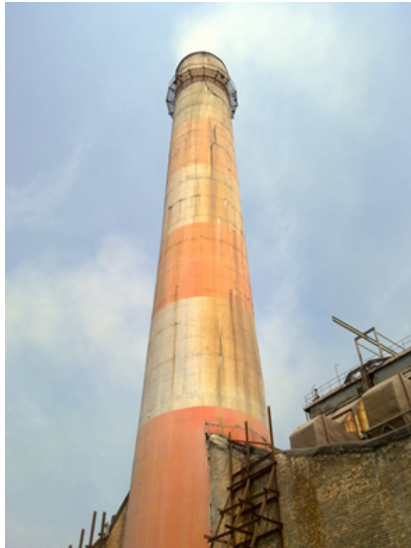
Figure 1.3: Single Flue RCC Chimney
