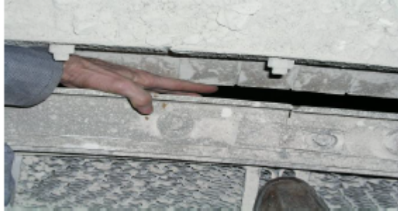
Figure 2.11: Original Circumferential Seal[21]
