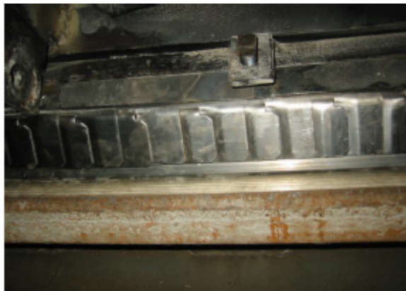
Figure 2.10: DURAFLEX Circumferential Seal[21]
