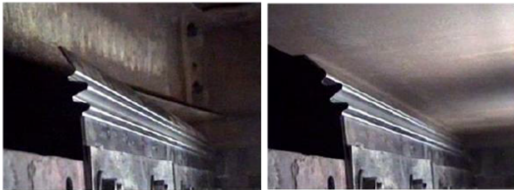
Figure 2.9: Continuous Contact DURAMEX Seal[21]
