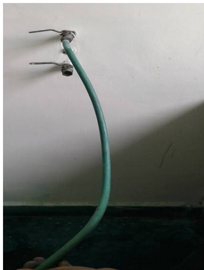
Figure 4.53: Air purging set up
