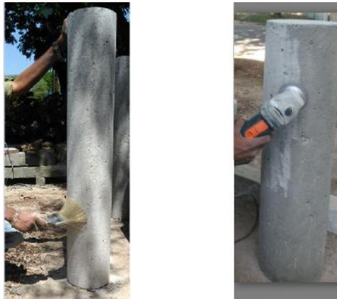
Figure 3.25: Cleaning of Surface and Grinding of Column
