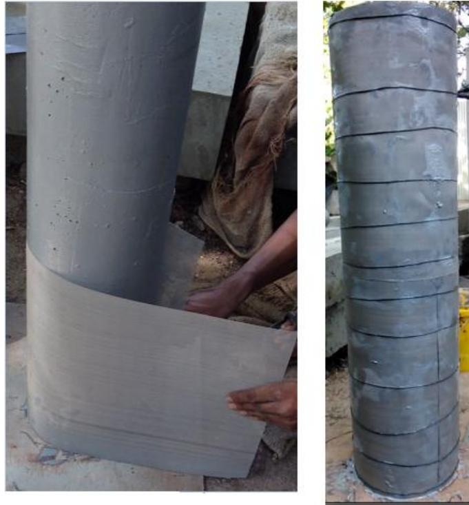
Figure 3.28: Wrapping of Mesh and Binding of Mesh
