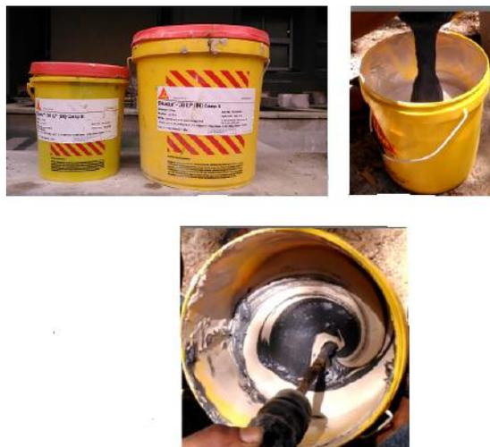
Figure 3.26: Mixing of material
