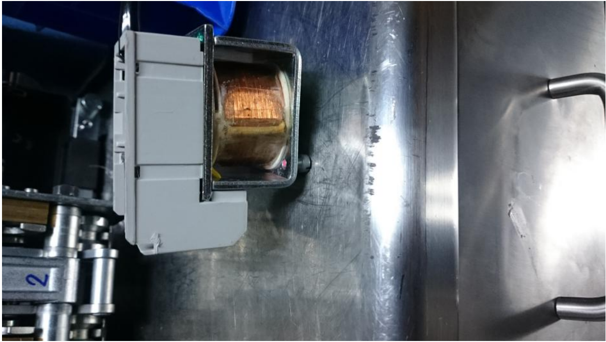
Figure 4.6: Trip Coil of single phase UVR
