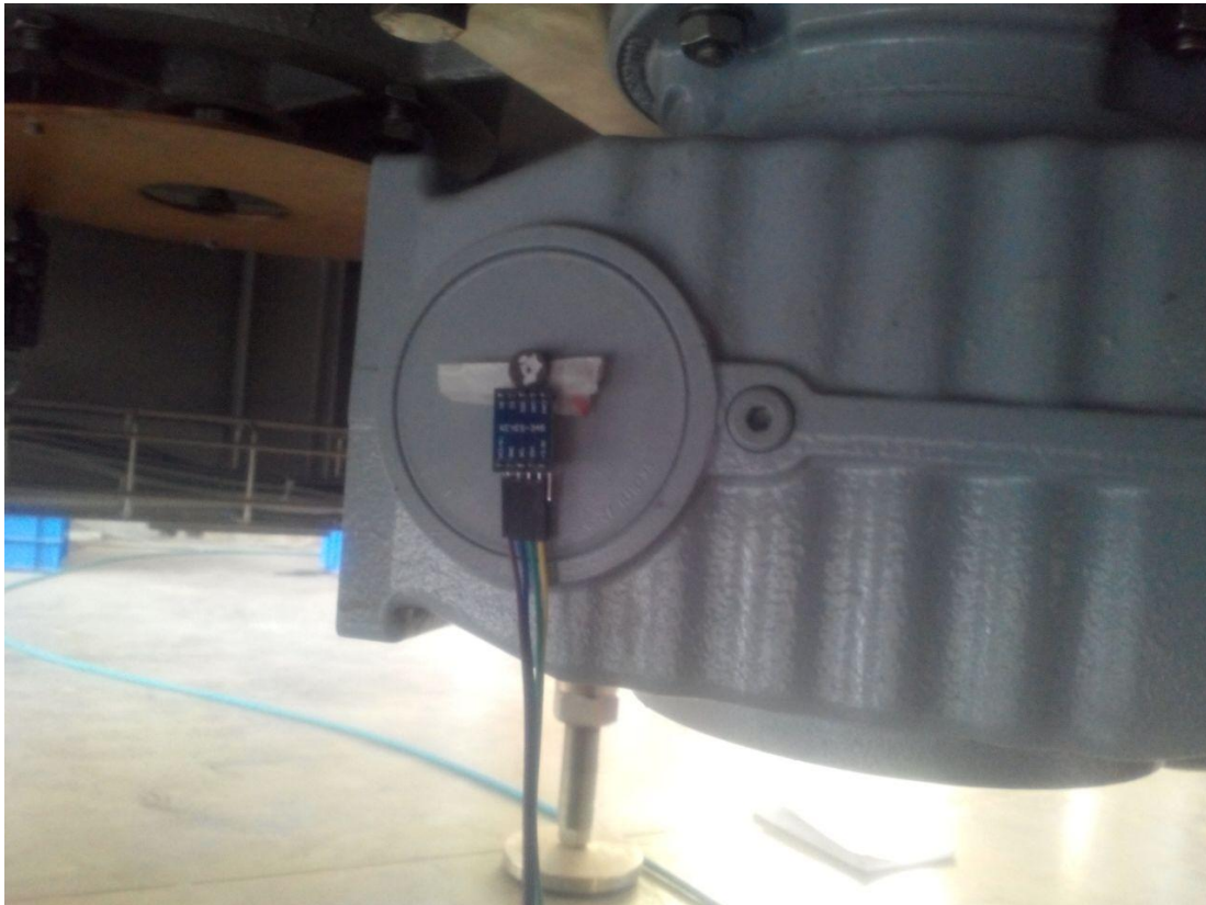
Figure 3.10: Mounting of Accelerometer on Gearbox
