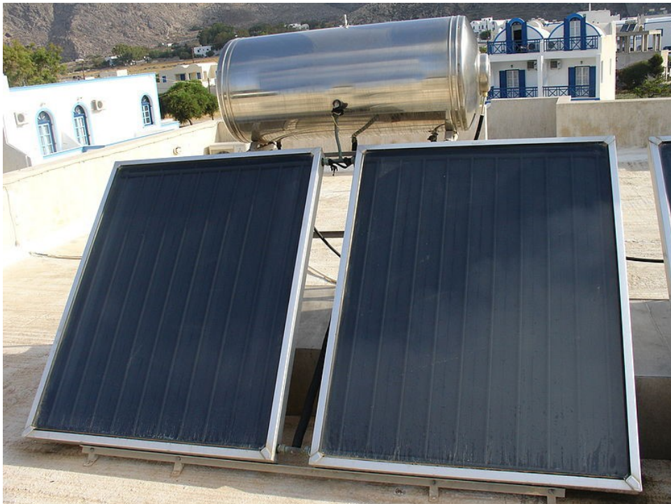
Figure 1.1: Flat plate thermal system for water heating [1]
