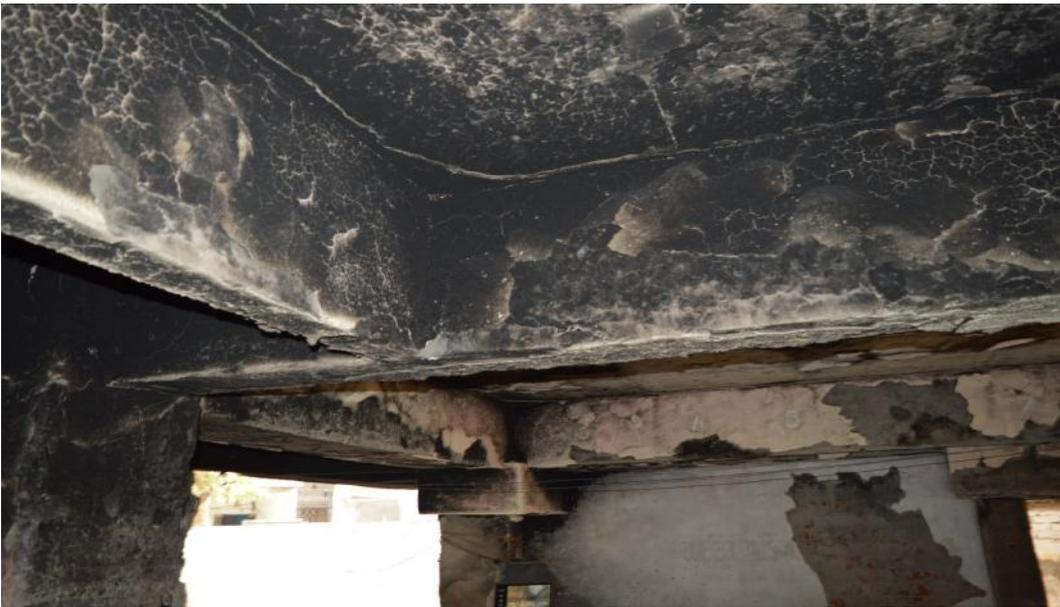
Figure 1.2: Damage Due to Fire (Saket Apartment,Ahmedabad)
