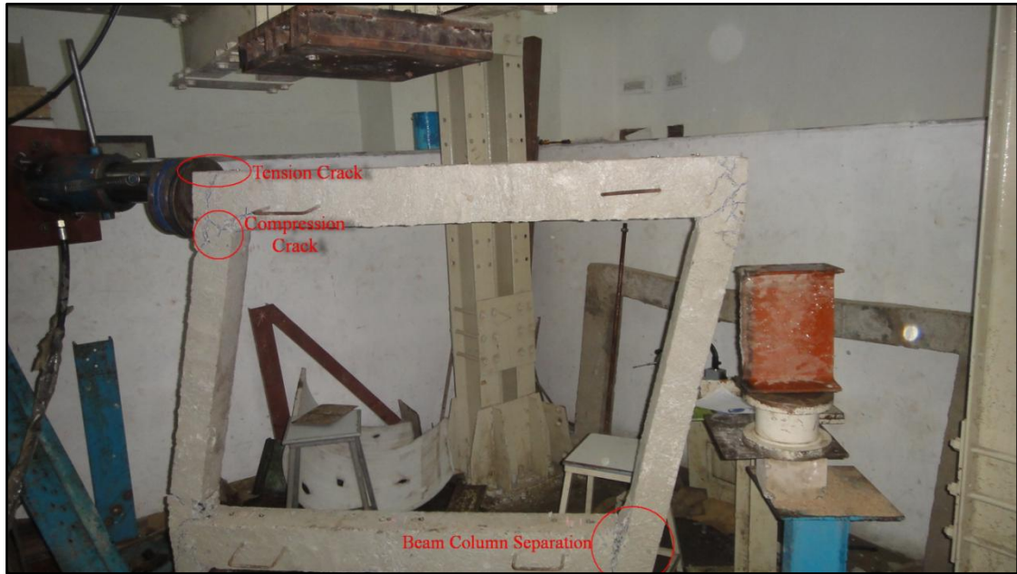
Figure 7: Failure in bare RC Frame
