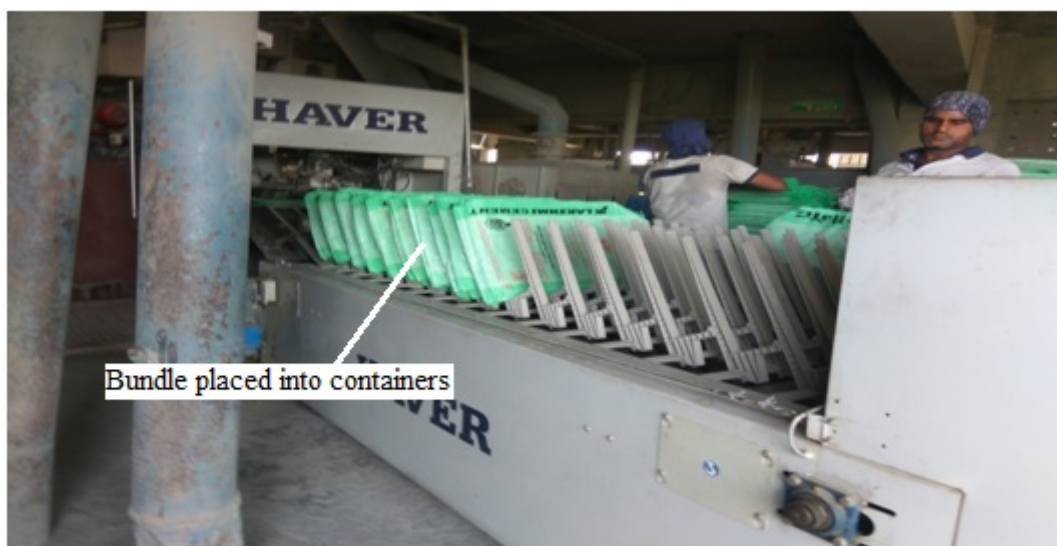
Figure 1.6: Automatic bag guiding machine with manual loading [ Courtesy: JK Lakshmi Cement ]
