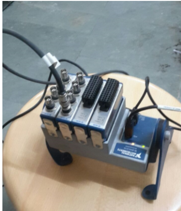
Figure 5.10: Data Acquisition System
