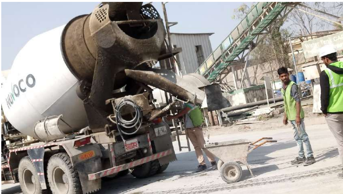
Figure 3.3: Collected Concrete Mix From RMC Plants
