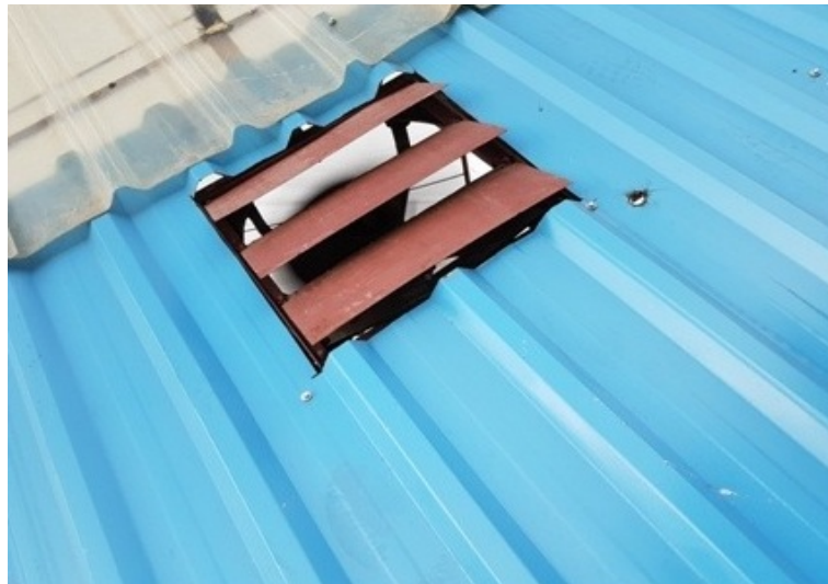
Figure 4.10: Fan - Louver system
