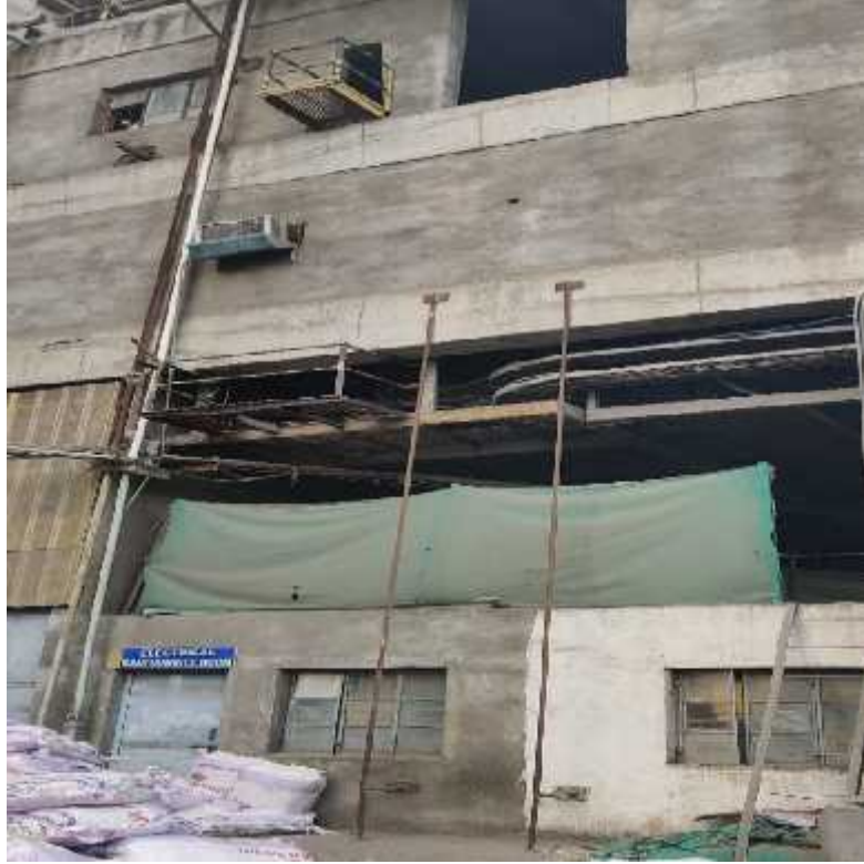
Fig. 1.4 Outside View of Bag Storage Area-1
