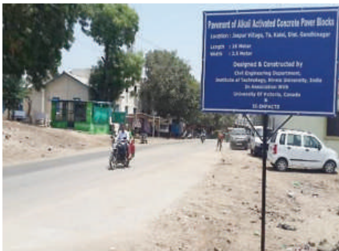
Stretch of Pavement using Paver Blocks of Alkali Activated Concrete at Jaspur Village, Dist. Gandhinagar
